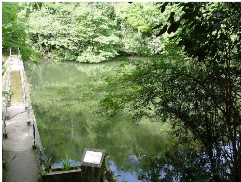
Figure 5: Epaminondas Ramos dam. (Aniszewski, 2009).
